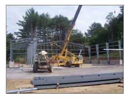
crane barely exceeded the height of nearby trees, we posted a NOTAM for a 110 foot crane, 600 feet east of runway 18/36 while the heavy construction was underway.
