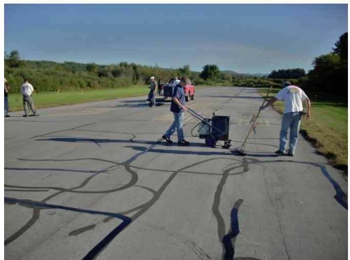
The crew seals cracks on Runway 18-36. Photo by Rick Kloeppel.
