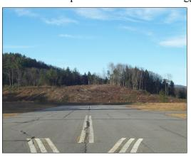
removing all trees that penetrate the 20:1 approach slope surface in a trapezoidal area 500 feet wide at the airport end and 1068
