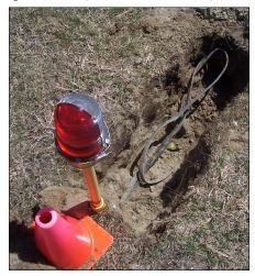
quadrant. Late last winter, the red circuit in the northeast quadrant failed, followed a couple of weeks later by the companion black circuit. Typically, our runway light circuits fail when water enters an underground connection that is
