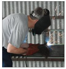
Following a period of inactivity over the winter, work has begun anew on the Parlin Field Hangar. **Terry Callum** is fabricating the structures necessary to support a new hangar door. The new structures will carry the load imposed by
