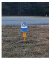
The lights have three levels of intensity: low, medium and high. Set on low, the lights perfectly mark the entrance of the mid-field taxiway. The LED lights are set to go on automatically from dusk to dawn. We will be purchasing two more to mark the entrance of the north taxiway. The simple stake mounted installation is a breeze and requires no trenching, wiring or electrical vault. So easy even our management could do it!
