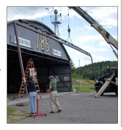
in place with help from a crane and operator provided by **LaValley Building Supply**. Once the frame was in place, Terry bolted and welded the frame to the existing hangar structure. The frame will provide the structural strength necessary to support a new one-piece hangar door.
