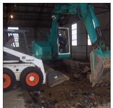
Over the past month, Jim and Terry Callum, with help from Mario Cusanelli and others, removed asphalt paving from the inside of the hangar. The old asphalt ranged from 2 inches to nearly a foot thick
