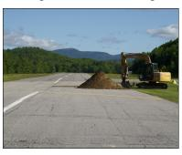
After consultation with Town officials, the airport hired a contractor to excavate the runway over the culvert to determine an exact cause of the failure. The excavation showed that significant
