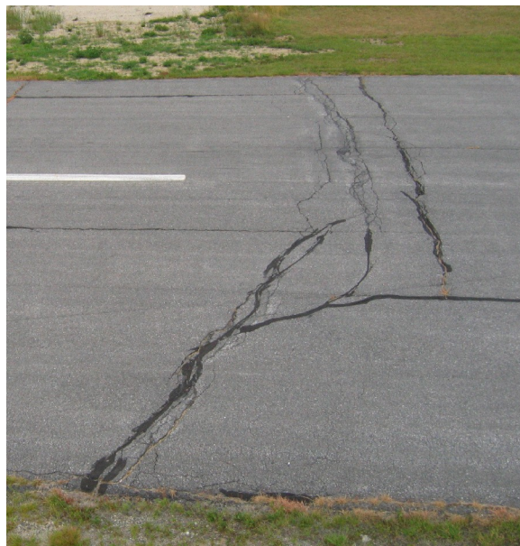
Illustration 2: Pavement rating POOR, wide cracks less than 50 feet apart with significant deterioration, settling, and deformation along crack edges.
