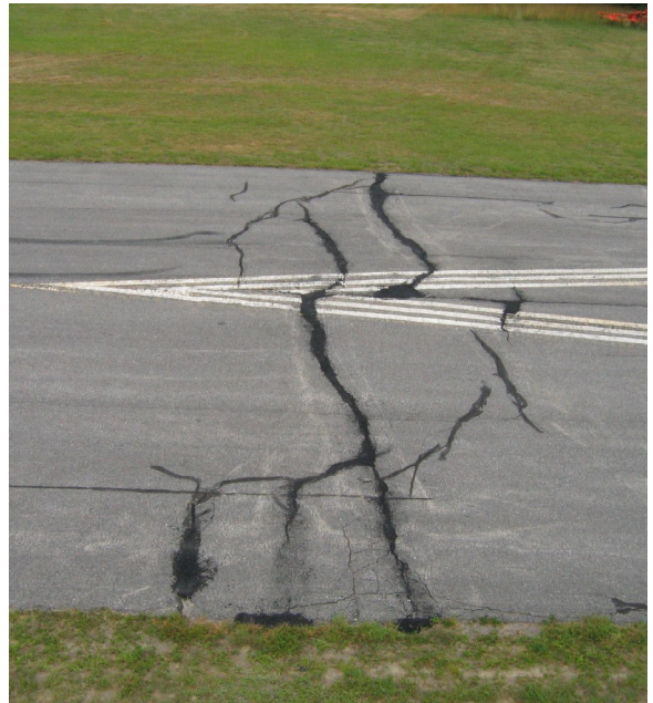
Illustration 4: Pavement rating POOR. Wide cracks with deterioration along crack edges and minor settling.
