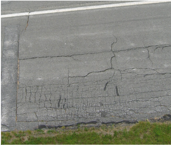
Illustration 3: Pavement rating POOR. Extensive alligator cracking over less than 20% of area, settling of 1 to 2 inches, and deformation.
