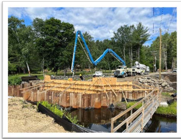
Pouring North Abutment Stem Wall
