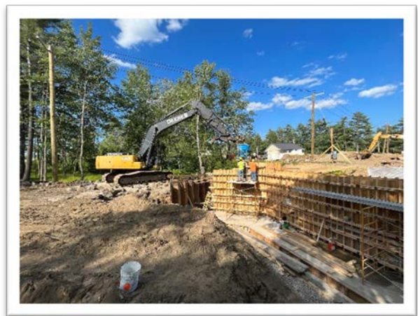
Pouring Northeast Wingwall
