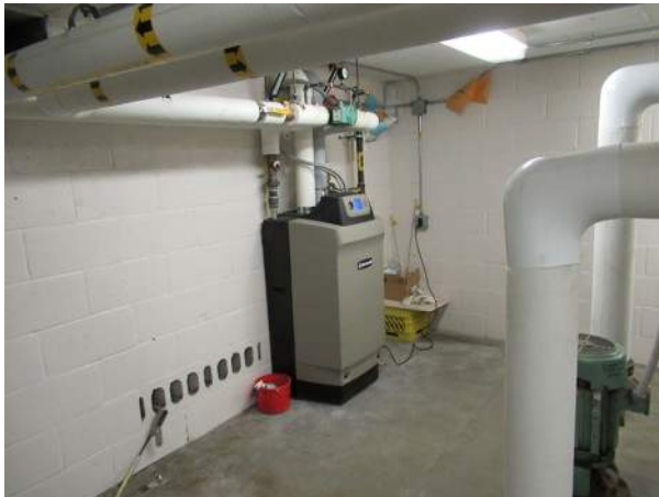
Photo 146—basement mechanical room, looking east at propane boiler.
