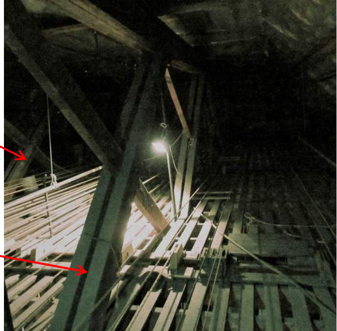
Photo 70—Two roof trusses that support roof of 1904 addition, looking north.
