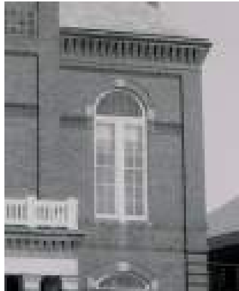
Photo 13 – Enlargement of Photo 12 showing half-round sash and satin glass prior to removal.
