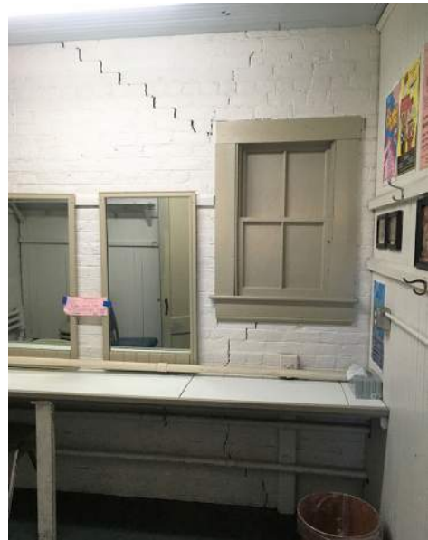
Photo 77 —Open mortar joints in west wall of dressing room in south west corner of mezzanine level.
