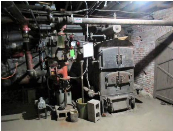
Photo 81 — North center of basement looking north, sprinkler system to left and old boiler (discontinued) at right.
