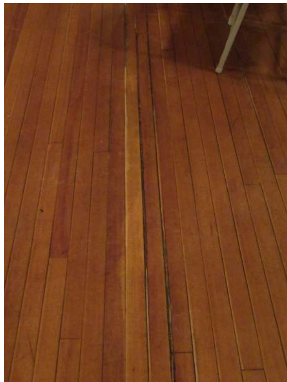
Photo 126— Example of split floor boards in Opera House
