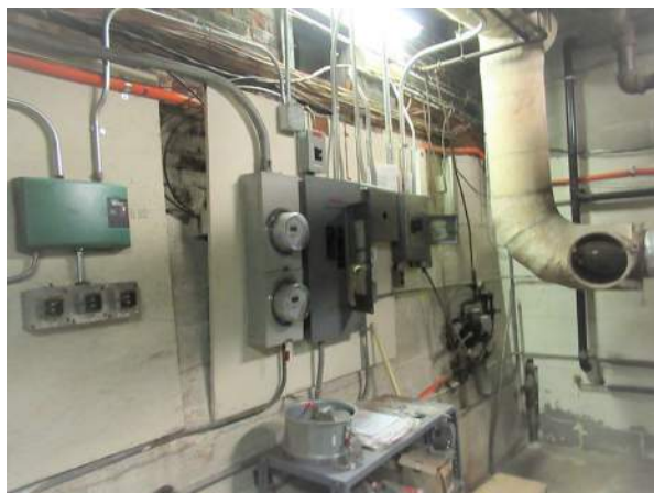
Photo 150— Electrical panel, meters and disconnects at east wall of first floor mechanical room.
