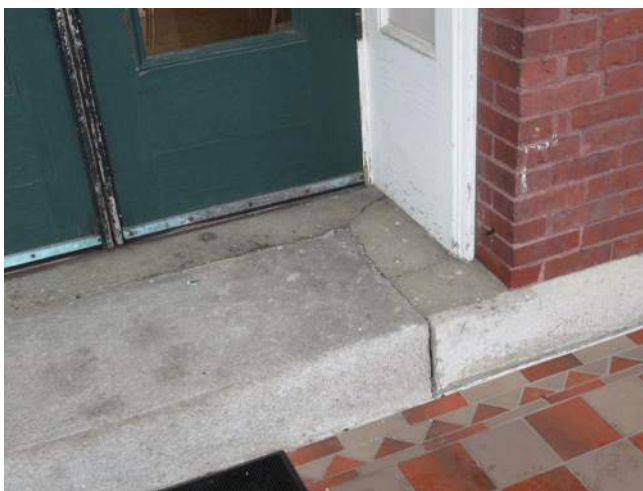
Photo 51 — Southernmost door at first floor main entrance at west side of building. Evidence that this entrance was altered in the past.
