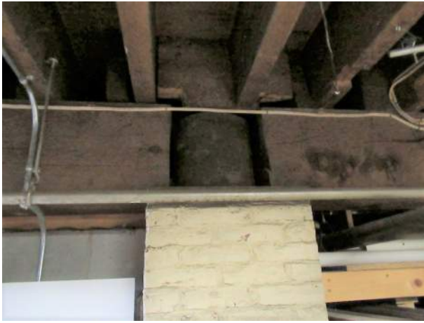
Photo 84 — Center of basement looking south at interior brick pier and base of one of the first floor steel columns.
