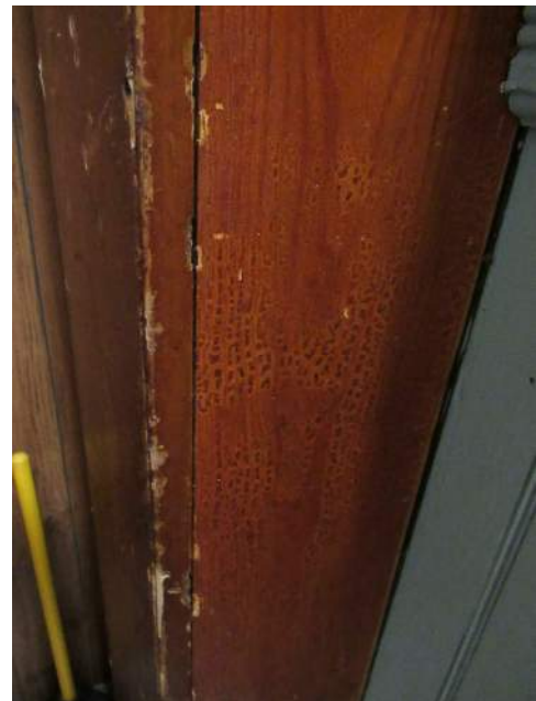
Photo 133— Example of clear finish with has 'alligatorated'.
