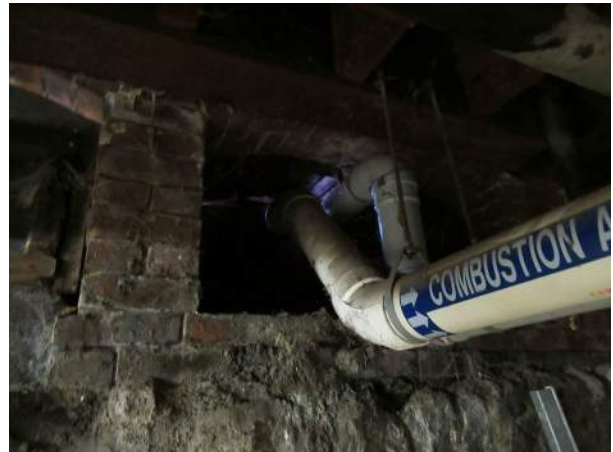
Photo 147—South exterior wall, vent pipe from propane boiler.
