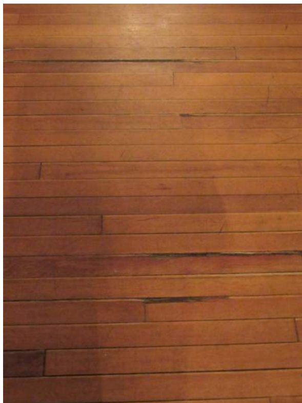
Photo 125— Example of split floor boards in Opera House
