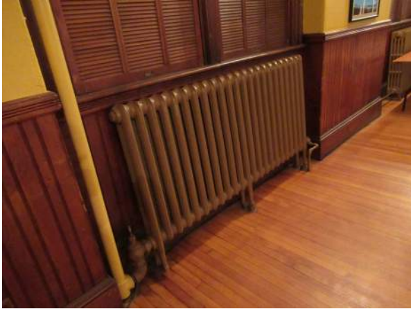
Photo 144—Cast iron radiator at north wall of opera house.
