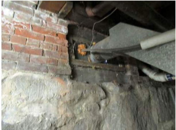
Photo 60 — South exterior foundation wall. The previous basement window openings seen here corresponds to exterior photo 50.
