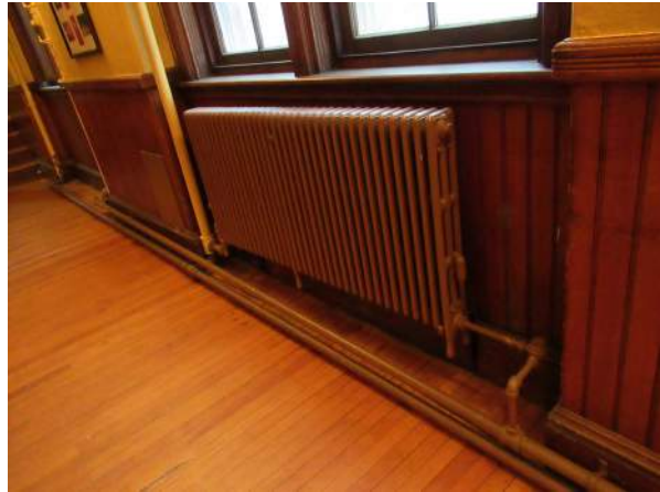
Photo 145—Cast iron radiator at south wall of opera house.
