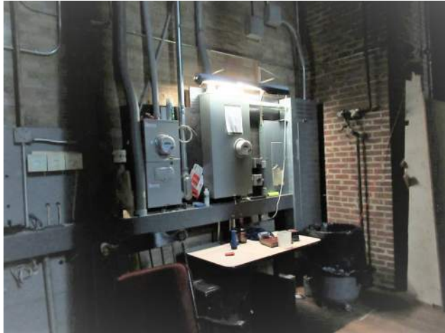
Photo 148— Electrical service, and meters at north wall of stage.
