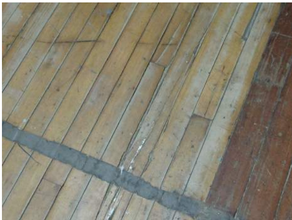
Photo 131— Example of split & cracked floor boards at stage.
