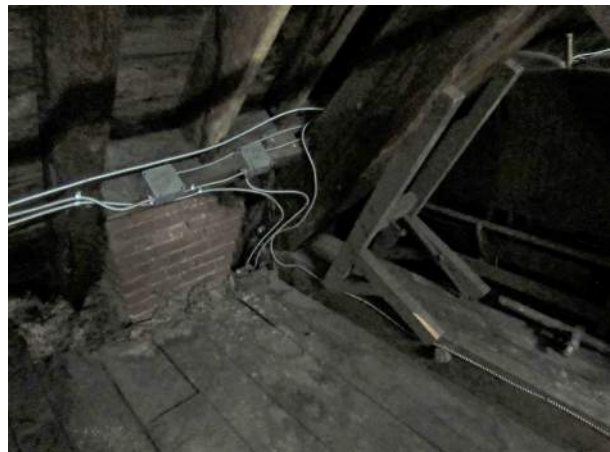
Photo 151— Example of wiring upgrades made in attic, at south exterior wall.
