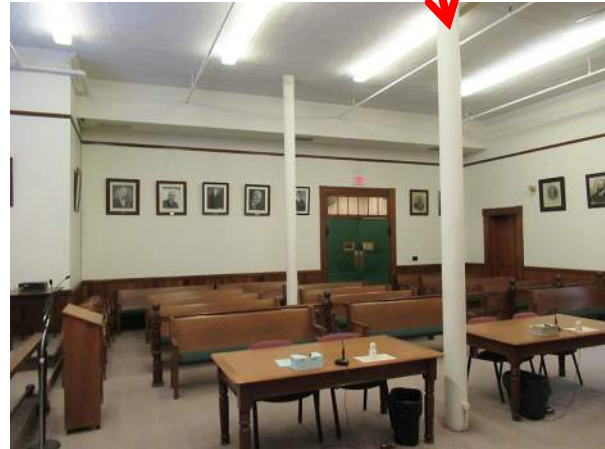
Photo 63—First floor court room looking west, two cast iron columns
