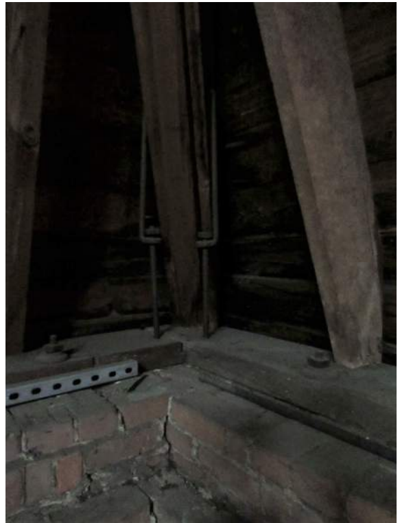
Photo 74—Close up of north east corner, note open brick joints
