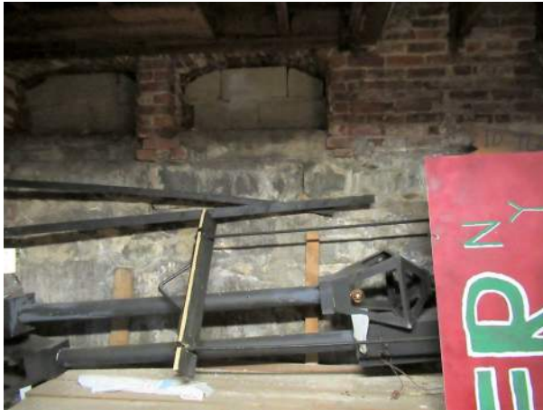
Photo 59 — North exterior foundation wall in basement, original basement windows in-filled with concrete masonry units, most likely when 1986 Courthouse Annex was constructed.
