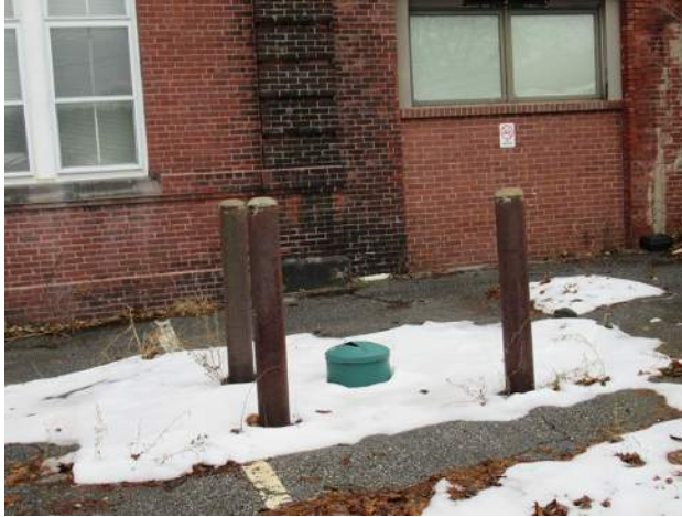
Photo 27—Cap for buried propane tank and protective steel bollards adjacent to south side of the building
