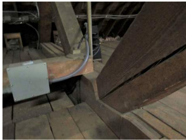
Photo 69—Top of south center steel rod supporting balcony at bottom of roof truss, looking south.
