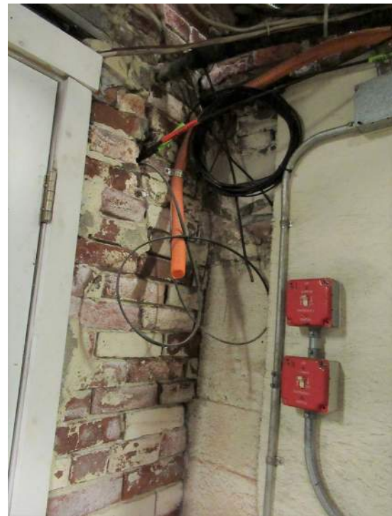
Photo 92 —North east corner of mechanical room showing deteriorated mortar joints.
