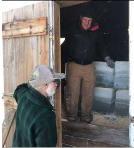
Packed in ice house [note sawdust insulation]
